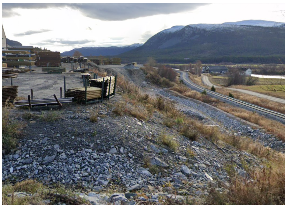
Figur 11: Steinmasser i fylling (Google maps)
